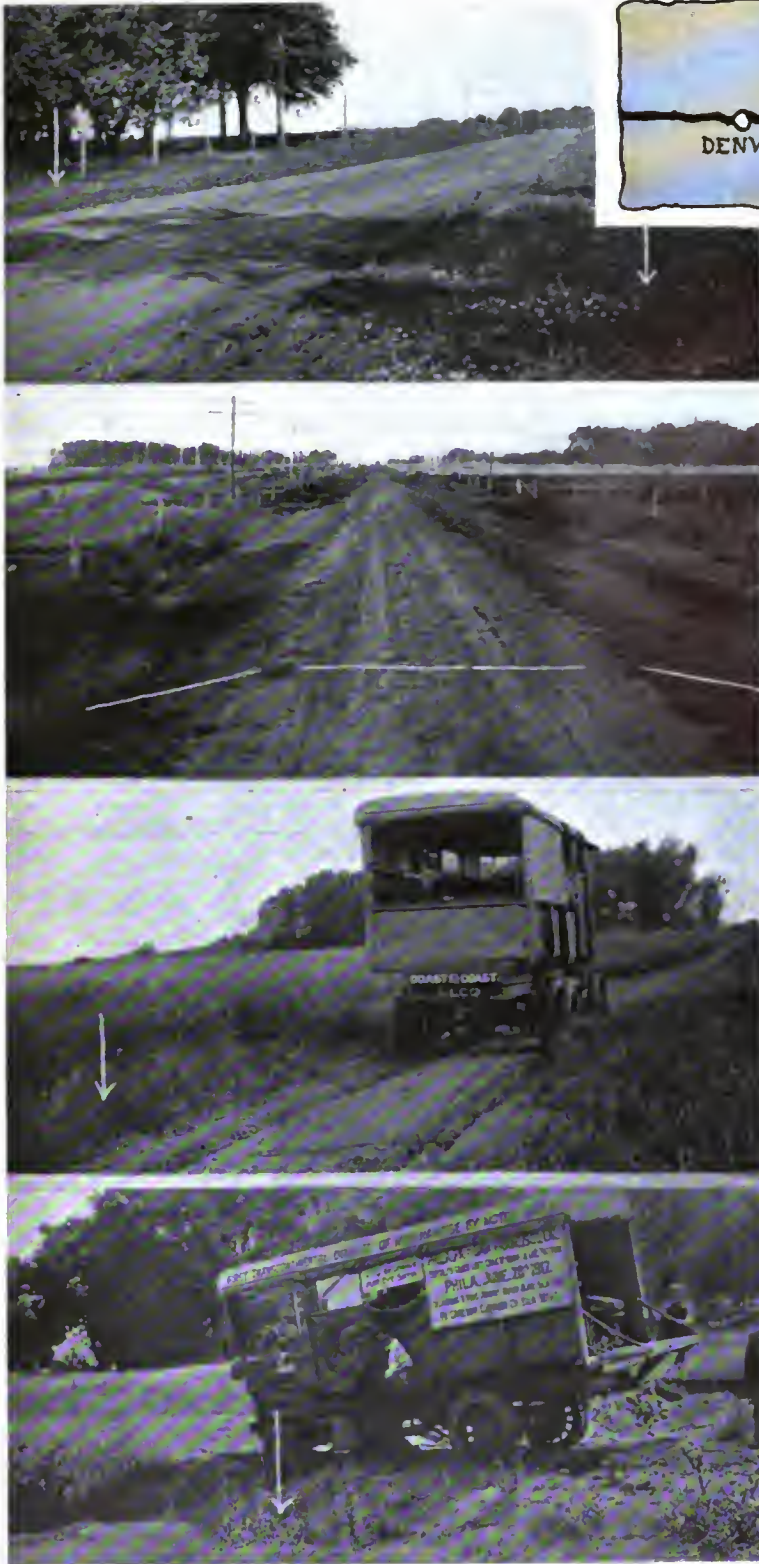
Top—Well-graded and slightly crowned, this road, near Marshalltown, Ia., has its surface maintained by dragging after each rain. Its one fault is that the side growth of weeds and grass should have occasional right-angle gutters that the surface water may flow to the shallow ditches on each side indicated by the arrows.
